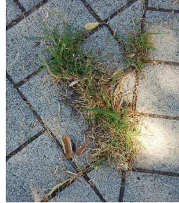
During the visual inspection, find locations with puddles or surface runoff that indicate possible clogging. Areas observed to have soil in the joints or vegetation growing in the joints indicate even more severe clogging problems. The probable causes of clogging (e.g. drainage from pervious upslope areas, vehicle tracking, wind deposition) should also be evaluated by your inspection team, to eliminate recurring problems and reduce maintenance needs.
