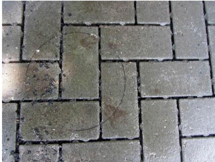
**Figure 6. PICP after two passes of the Cyclone machine. Note aggregate and sediment removed resulting in open joints.**
